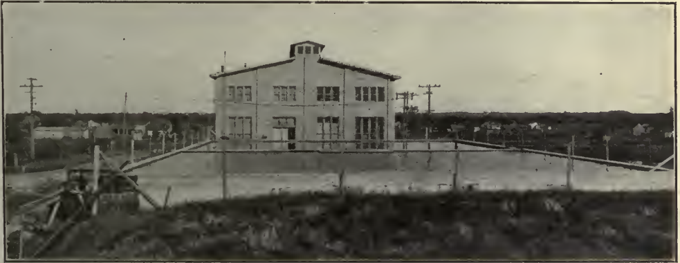
EXTERIOR OF MIAMI, OKLA., WATER-WORKS, SHOWING BASIN AND POWER-PLANT
